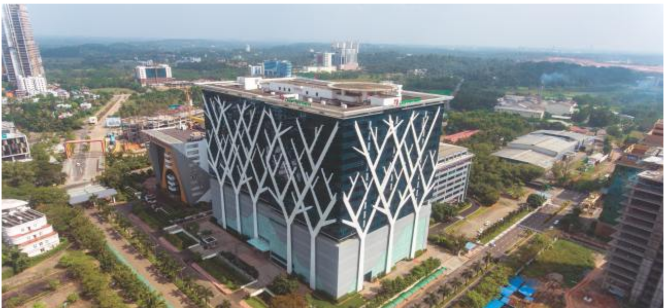
LULU Cyber Tower 2 - Single largest co-developer building (1.3 Mn Sq. Ft)
