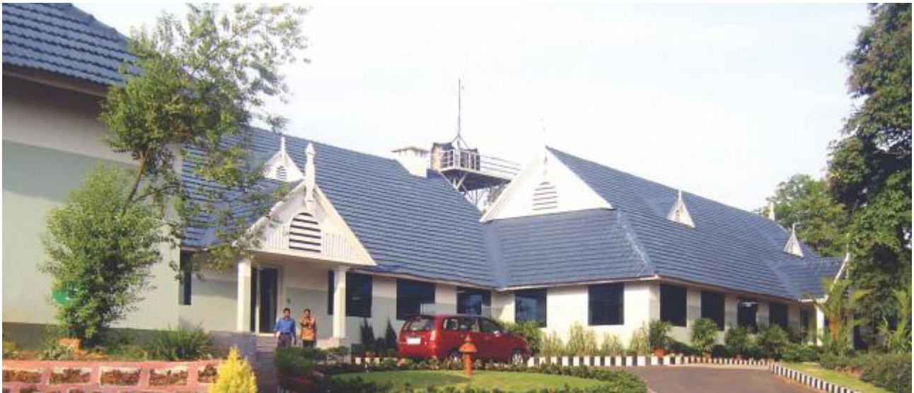
Villa Building - The traditional buildings renovated
